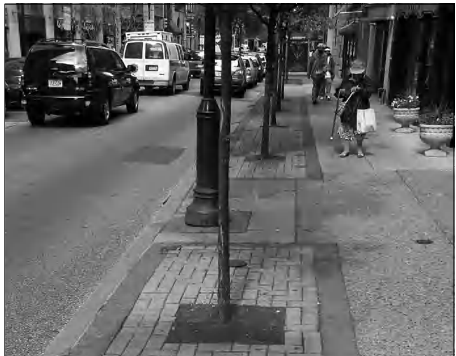
Large sidewalk cutouts and innovative planting design should be used for larger trees.
