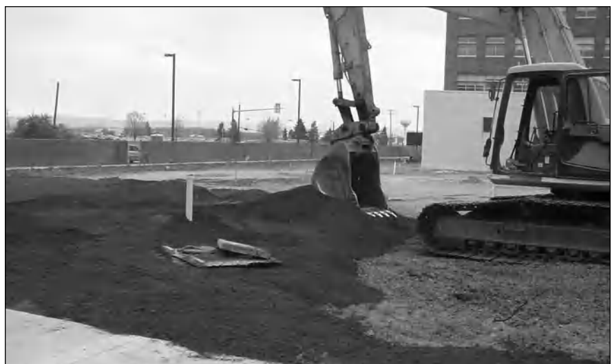
As shown in these three photographs, soil amendments are applied and cultivated throughout the planting area, not just the planting hole.
