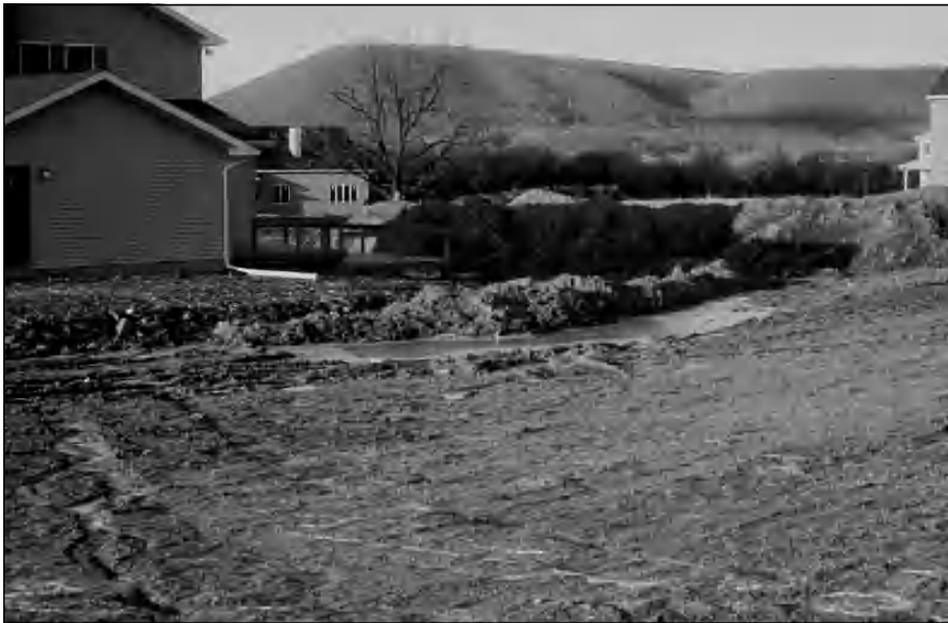
This soil's structure has been crushed and destroyed by compaction or mashed and destroyed by rough treatment.
