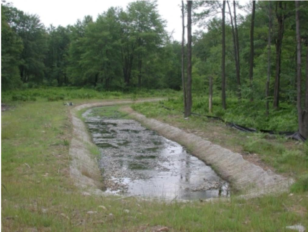
**Figure 3. An open channel utilized to aerate effluent from the Pebble Run Vertical Flow Wetland in the Mosquito Creek Watershed.**
