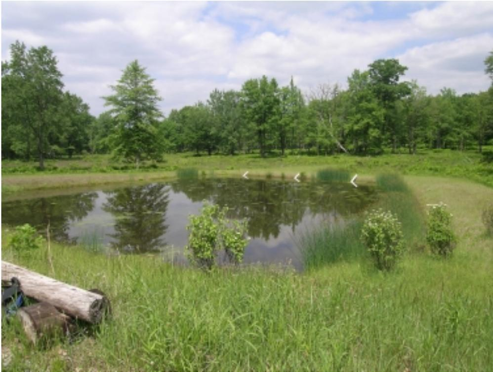
**Figure 2. The Ardell Road Vertical Flow Wetland System installed to treat acidic water in a headwater stream of the Mosquito Creek Watershed in Clearfield County. Water in this pond percolates through compost and limestone before discharging directly to the stream.**
