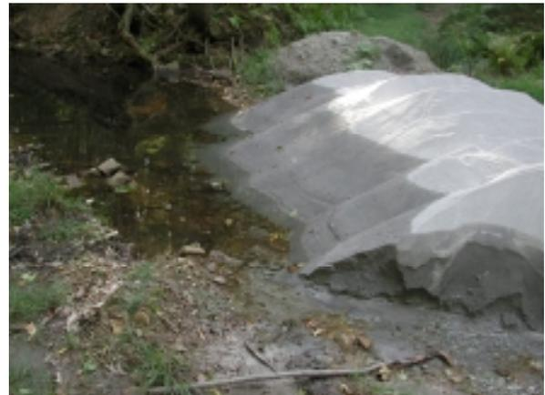
**Figure 2. Direct application of 25 tons of limestone sand to an acidified headwater stream in Westmoreland County.**
