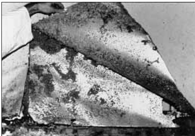
Figure 11. Destruction of insulation by litter beetles.
